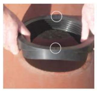
Make a clean, 90° core cut into the pipe wall using only a diamond core bit unit specified by Mission Rubber. Ensure there is no foreign matter or contaminants on the core surface, TwisTee stub-out (B) or the TwisTee rubber gasket (A).
