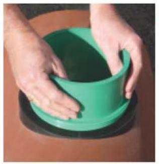
Place the TwisTee stub-out (B) into the TwisTee rubber gasket (A), ensuring the threads are properly aligned. Using both hands, slowly tighten clockwise until most of the threads are engaged.
