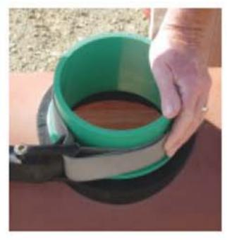
Place the strap wrench around the TwisTee stub-out (B). Tighten clockwise in a continuous motion until the top thread of the TwisTee stub-out (B) is flush with the
